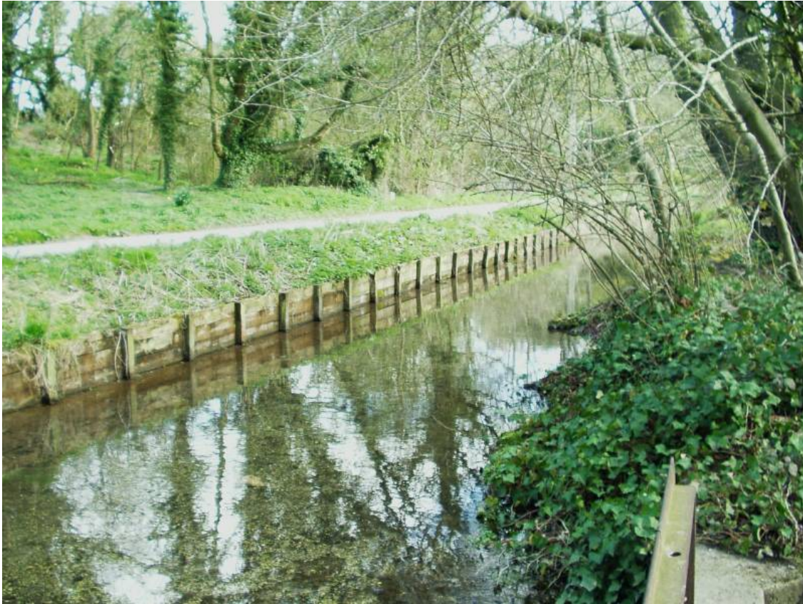
Illustration 7: Hard Revetments Along Tributary Channel
